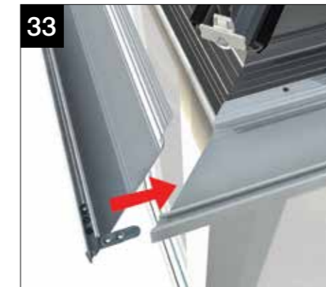
Fit the cleats (CRN001) to the desired side using the fixings provided (CRN006) as shown and assemble the remaining lower sections
