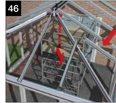
Now start on the jack rafters. The two part jack rafter kit will already be fitted to the hip and jack rafter bars. Again refer to the location plan and corresponding labels attached to the parts.
