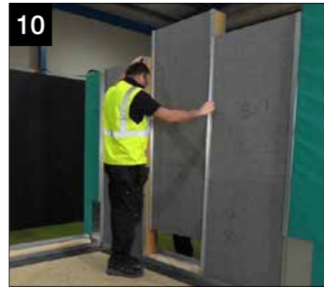
10 Lift the walling panels into place starting at the ends before filling in towards the middle.
