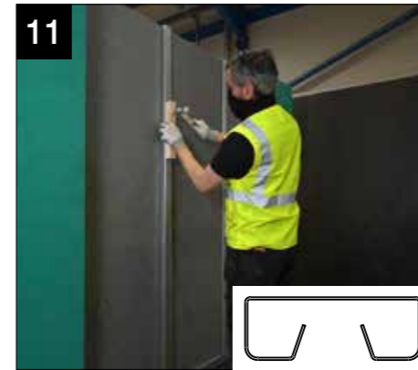
11 Secure walling panels together using the provided steel clips both internally and externally, these can either be pushed into place or slid down from the tops of the panels.
