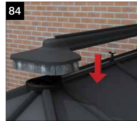
84 Offer up the complete ridge capping onto the roof.
