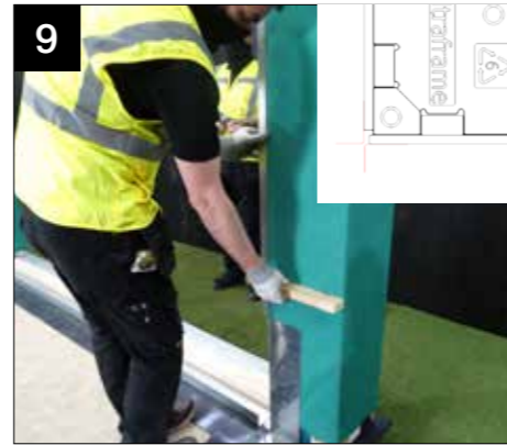
9 At the walled elevations align column to walling brackets to the edge of the column and to the top of the column structural bracket and secure to the column using NRTF050 (4.2 x 25mm wafer head screws) through the pre-punched holes.
