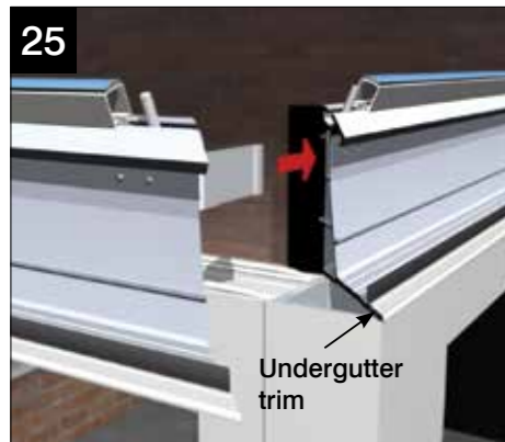
Prepare the cill that abuts the tall columns with the detail shown to accommodate the column claddings.
