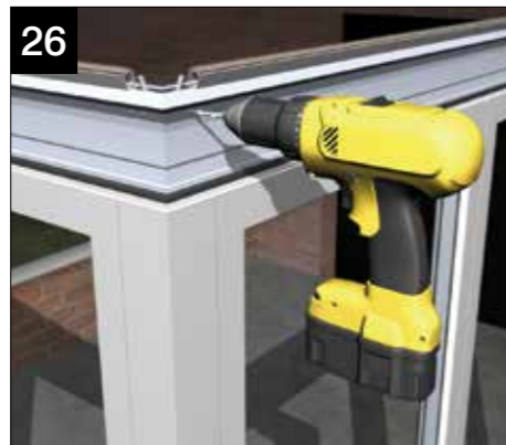
Using the pre-drilled pilot holes, drill two 4.5mm holes through the corner cleats.
