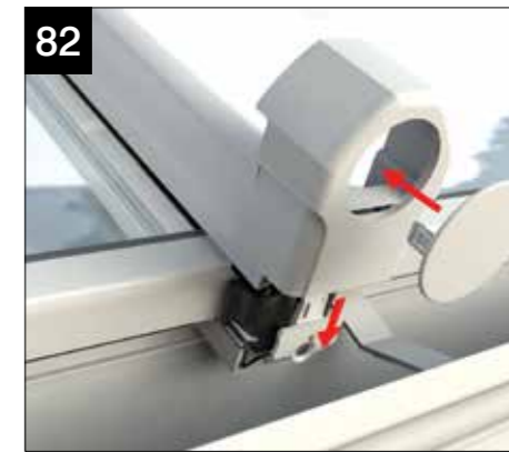
82 Fit the glazing bar end caps by sliding onto the fixing blocks. Push fit the insert into the end cap.
