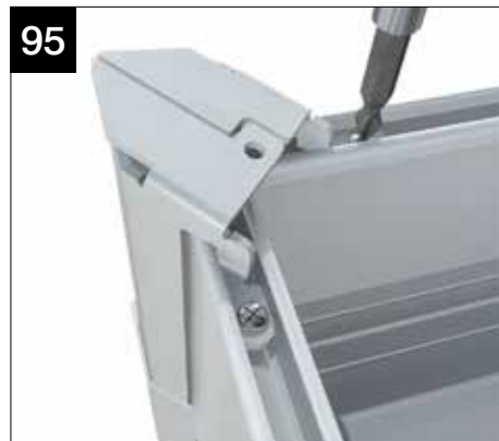
Whilst ensuring the corner remains in position, screw fix using CRN007.
