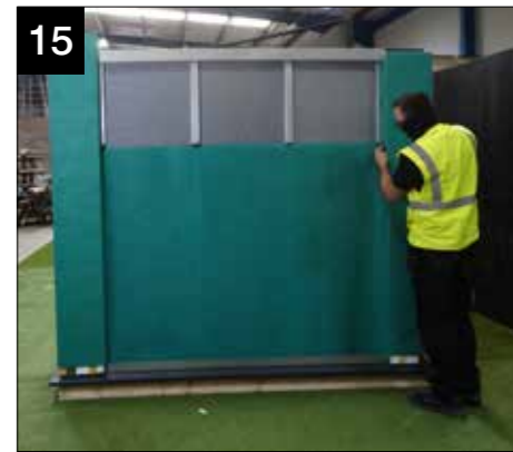
15 Using the provided roll of membrane, stretch out horizontally across the lower half of the wall and temporarily pin in place using staples or tacks into the corner columns. Repeat across the upper half of the wall overlapping the lower covered area. Repeat the process on all walls.
