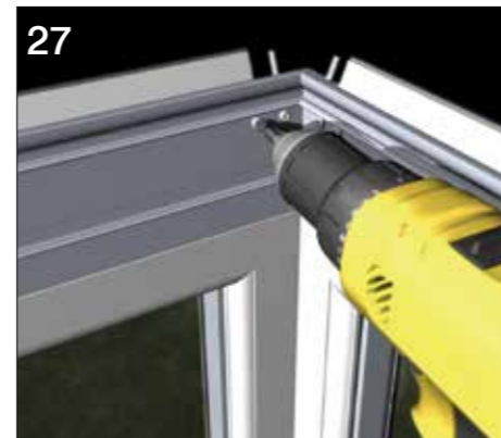
Securely fit the two M5 x 12mm tapite screws EBT001.
