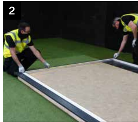
2 Evenly position cill on slab/base sealing any joints with an appropriate sealant. Check diagonals to ensure square and fix cill in place to aid positioning.
