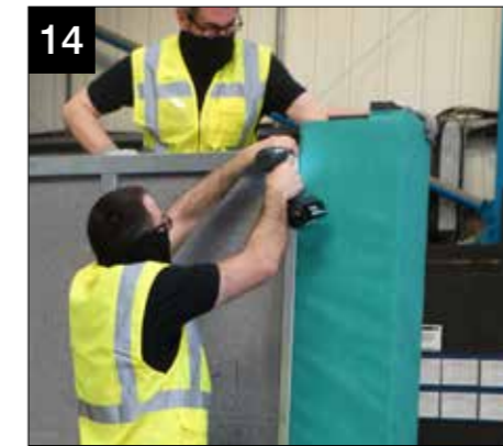
14 Secure the top tray to the interior wall panels through the pre punched holes using the supplied 13mm self drilling screws (CHAA006).
