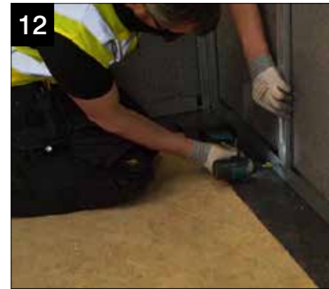
12 Ensure the walls are pushed against the internal steel of the base trays and fix in position through the pre punched holes in the base trays and column angle using the provided screws (CHAA006).
