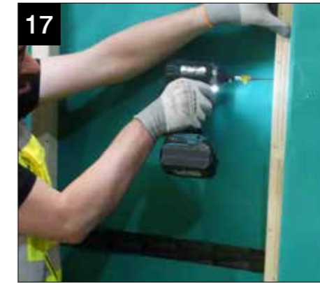
17 Starting with the clips closest to the columns, fix the battens to the columns using provided fixings (NRDS070), pushing the batten up against the underside of the top tray. The timbers can then be fixed into the walling panel clips using FSW-55-70/10 towards the top, centre and bottom of the timber batten.
