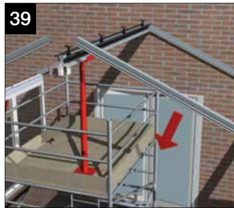
Continue to support the ridge and offer up the transom glazing bars (above), loosely attaching using the roofing nuts and bolts supplied. Ensure the rain baffle upper leg is lifted prior to placing the glazing bars.
