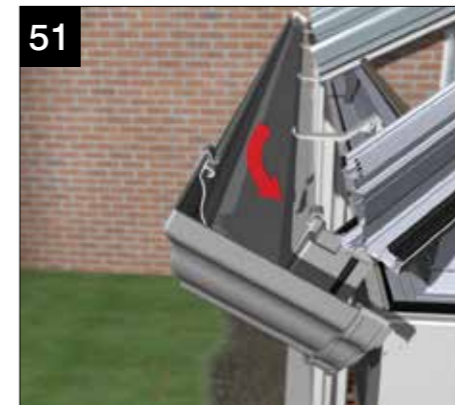
Locate the back edge of each section of gutter into the slot in the gutter bracket.
