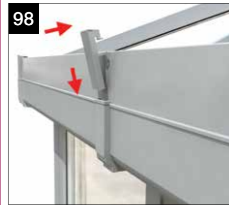
Slide the bracket into place ensuring bracket cleats slot into the top cornice section.
