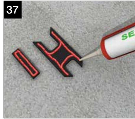
Take 'rubberised' sealer strips and generously butter with silicone.
