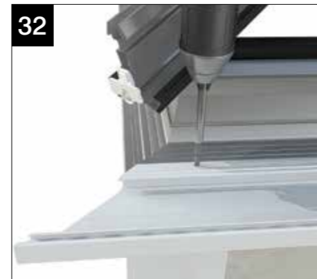
Prior to fitting gutter offer up the lower cornice section then secure into position using the fixings provided (CRN007). Please note: Always start with the front facet!
