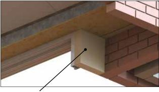
Infill 70 x 265mm In this case infill option is shown as timber.
