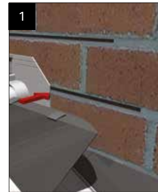
Apply 2 beads of silicone to integral weather-bars - insert into 35mm slot.
