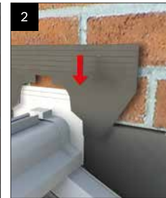
'Butter' with silicone and fit pre-cut saddle trim.
