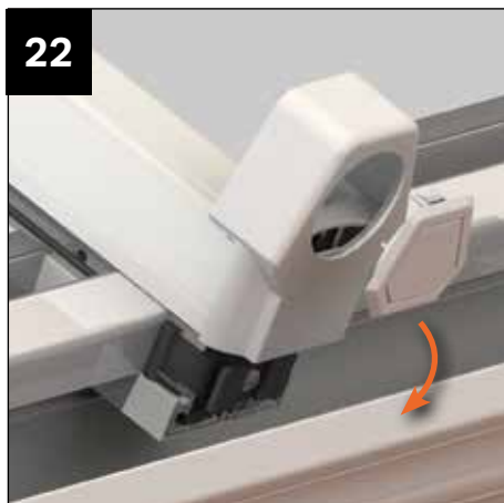
If you haven't fitted already, attach end cap fixing brackets. Fit the rafter end caps by sliding onto the end cap brackets. Push fit the insert into the end cap.
