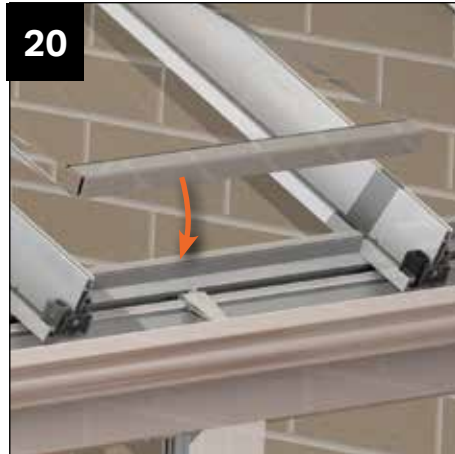
At this point the roof should be glazed. Any ridge support may be removed. Insert the glazing between the rafters ensuring that it is centralised.
